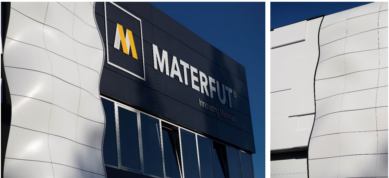
Materfut® headquarters, in Portugal. Facade with Corian® Exteriors panels (made with Corian® Solid Surface) showcasing different shaping possibilities, including organically shaped panels created with parametric design; Project by architect Alexandre Sousa Lopes; fabrication and installation by Materfut®; photo by Pedro Pinto for Materfut®, all rights reserved.
