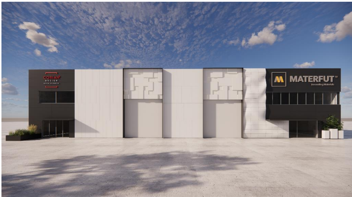
Materfut® headquarters, in Portugal. Facade with Corian® Exteriors panels (made with Corian® Solid Surface) showcasing different shaping possibilities, including organically shaped panels created with parametric design; Project by architect Alexandre Sousa Lopes; fabrication and installation by Materfut®; Image by Materfut®, all rights reserved.
