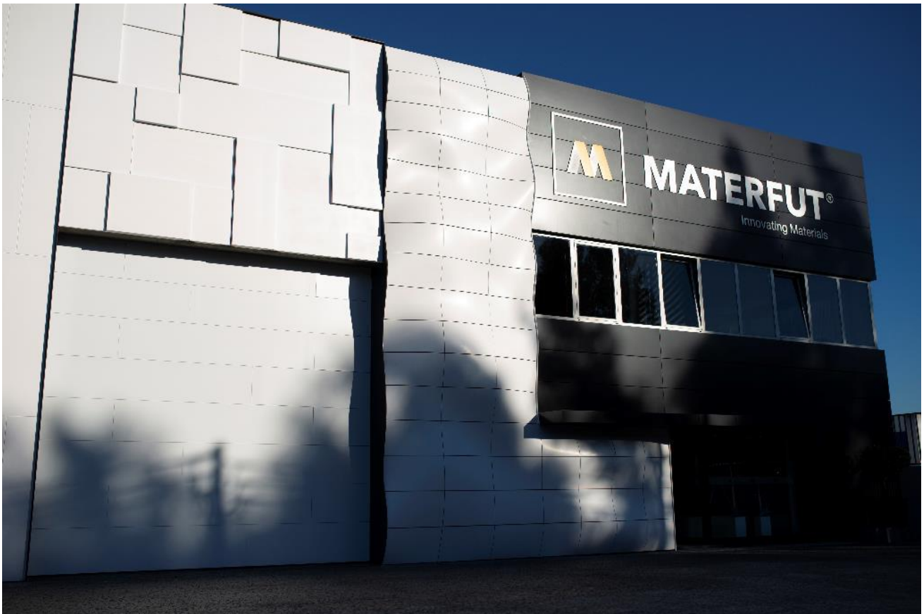
Materfut® headquarters, in Portugal. Facade with Corian® Exteriors panels (made with Corian®Solid Surface) showcasing different shaping possibilities, including organically shaped panels created with parametric design; Project by architect Alexandre Sousa Lopes; fabrication and installation by Materfut®; photo by Pedro Pinto for Materfut®, all rights reserved.
